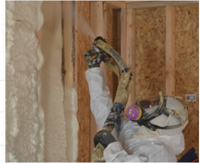
Spray Foam Insulation
