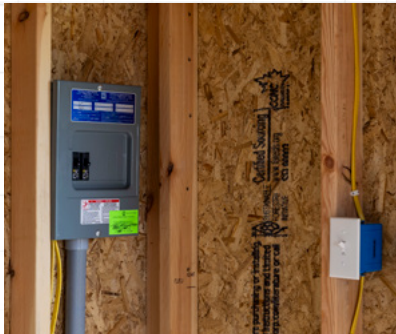
Electrical Packages Installation
