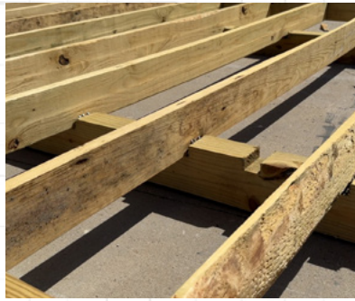
12" on center Floor Joists
